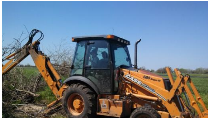
Jerry & Matt Boone running the backhoe
